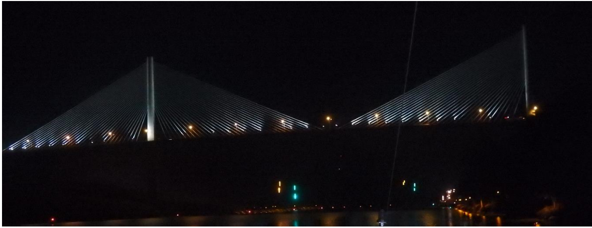
Centennial Bridge after clearing the last locks and entering Lake Gatun
