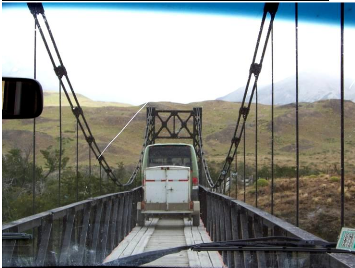
Remove external mirrors before crossing bridge!
